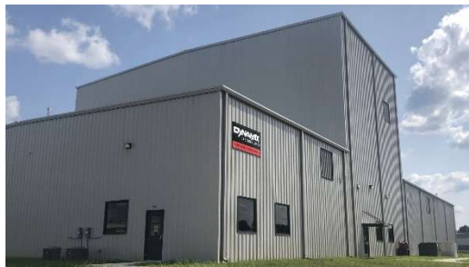
Dynamix Plant located in Huntingdon, TN
