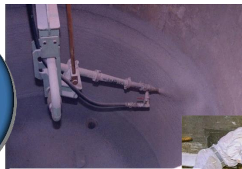
Furnace Construction Division
