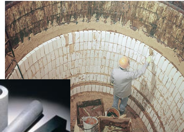
Furnace construction using fire bricks
