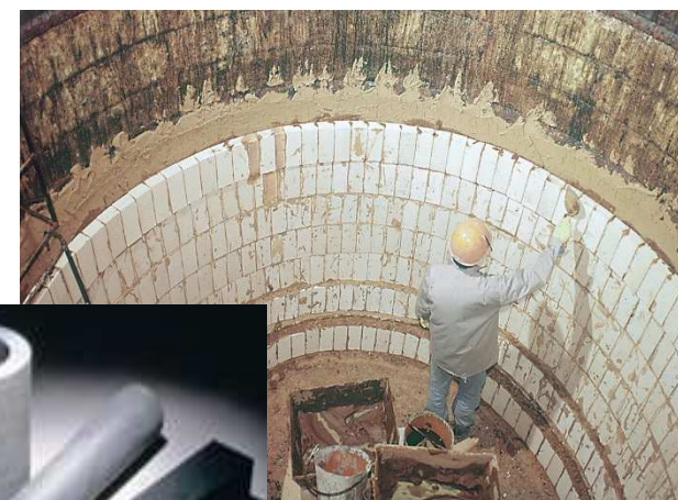
Furnace construction using fire bricks
