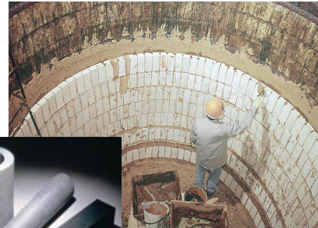
Furnace Construction using Fire Bricks
