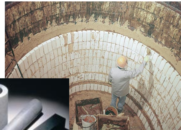
Furnace Construction using Fire Bricks
