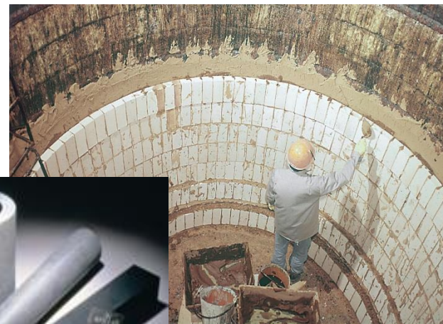
Furnace Construction with Fire Bricks
