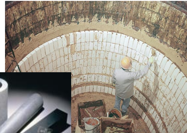
Furnace Construction with Fire Bricks
