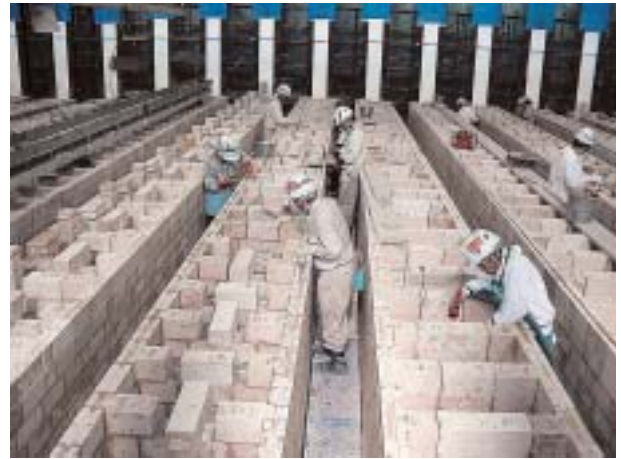
Fig. 2 Coke oven brick laying. (Part)
