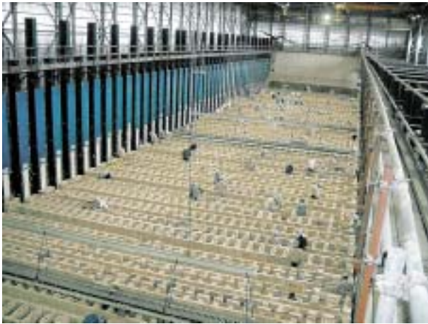
Fig. 1 Coke oven brick laying. (Whole)
