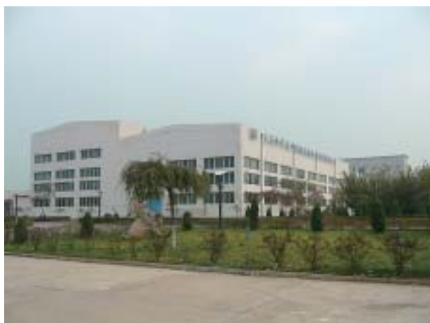
Fig. 1 Appearance of plant.
