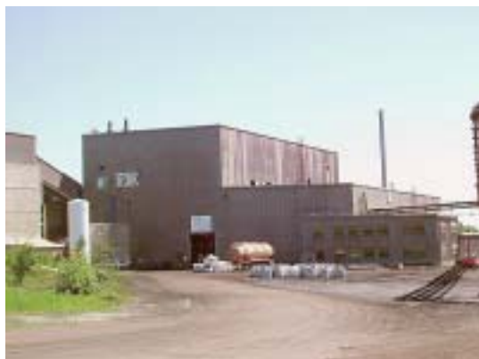
Fig. 7 Demonstration Plant in Minnesota.
