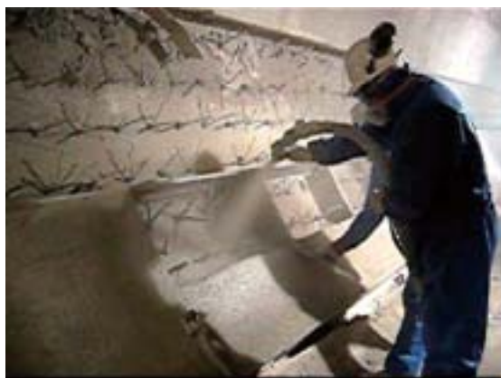
Fig. 5 Gunning in the Rotary Kiln.
