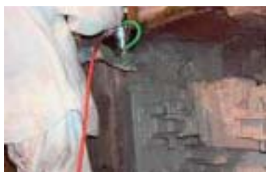
(a) Applying WALL-GUARD
