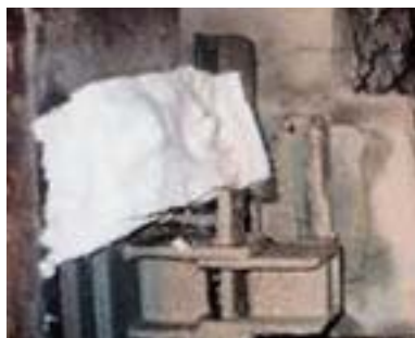
(b) After WALL-GUARD being gunned
