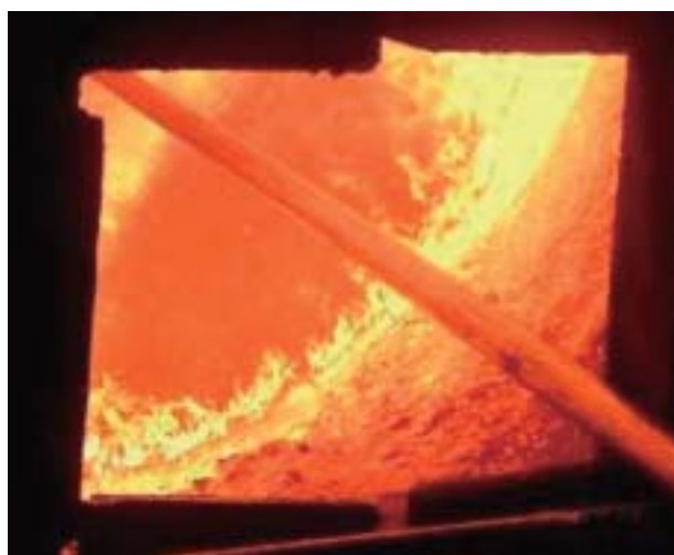
Fig. 1 Gunning on inner wall of BOF in hot condition.
