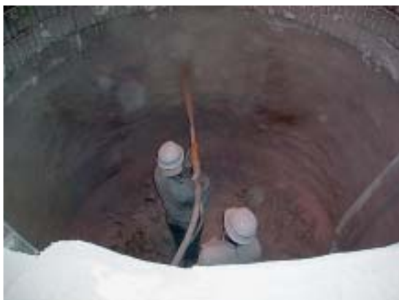
Fig. 1 Condition of gunning.
