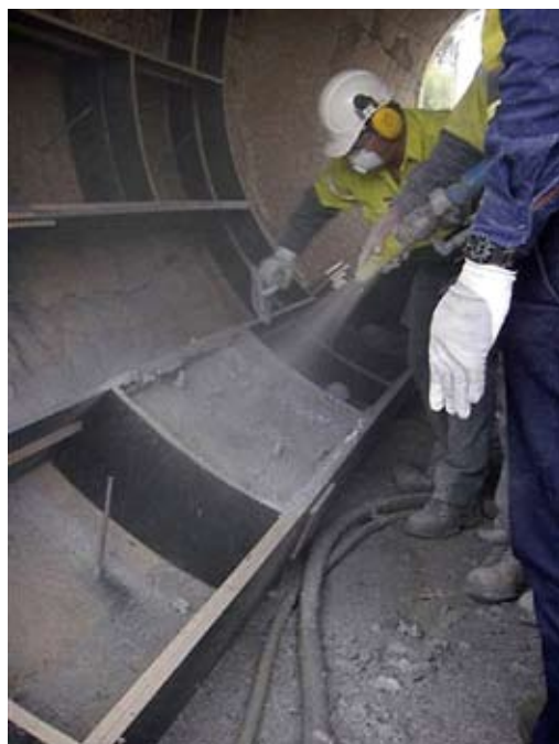
Fig. 1 CLEANSHOT 60M installation trial.
