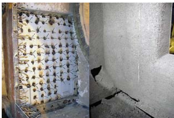
Fig. 3 Before and after installation of CLEANSHOT ZS at cooler-cement kiln.
