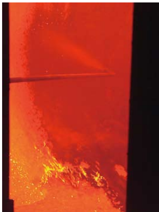
Fig. 1 Gunning on inner wall of BOF in hot conditions.
