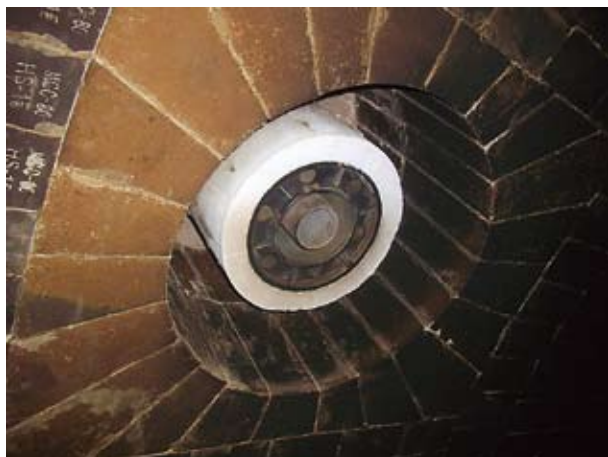
Fig. 5 Setting of gas burner in the ceiling.
