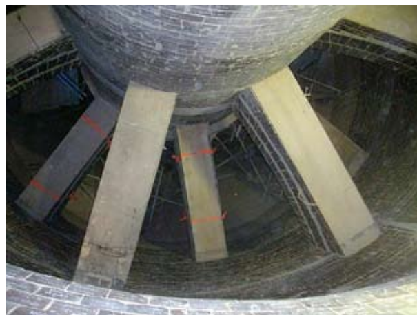
Fig. 6 Arch structure to support the center column.
