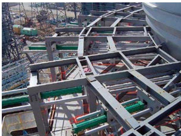
Fig. 3 Arrangement of pushers.
