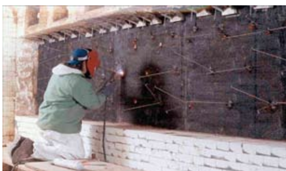
Fig. 5 Anchor welding
