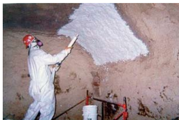
Fig. 8 Foamfrax gunning
