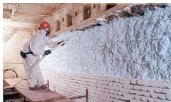
Fig. 6 Foamfrax gunning
