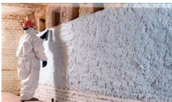
Fig. 7 Surface trowing
