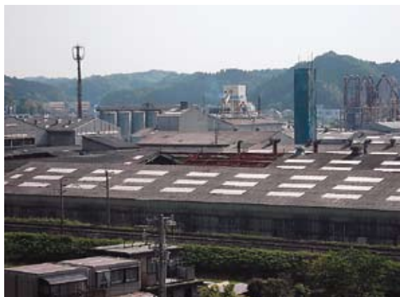
Fig. 4 A distant view of plant under recovery construction.
