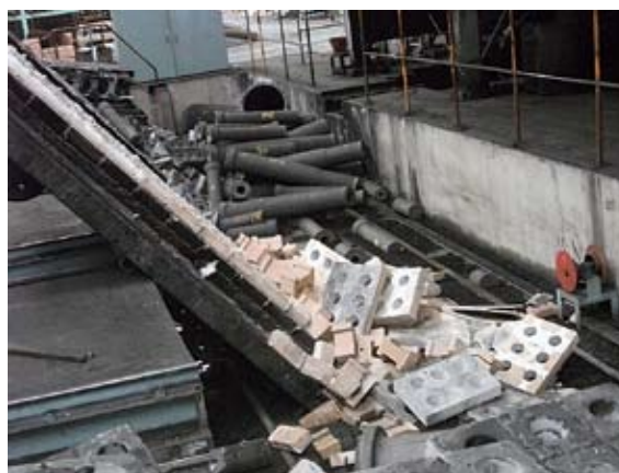
Fig. 3 Kiln car which fell down into traverser pit.
