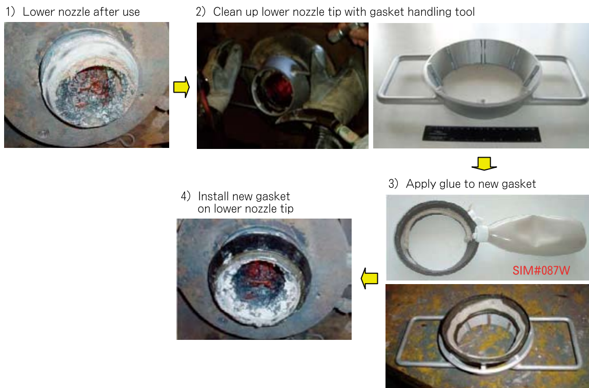
Fig. 3 Installation procedure for lower nozzle gasket.
