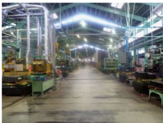
Fig. 1 View of plant after remodeling.
