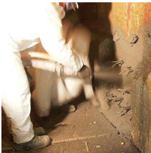
Fig. 6 Installation of NOVACRETE® product.
