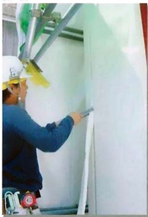
Fig. 5 BSSR blanket as fire protection of building. BSSR is used as joint sealer.
