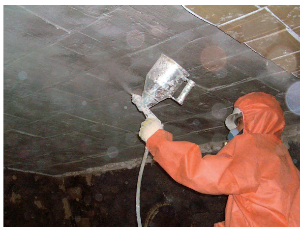
Fig.6 Spraying coating product on the hot face of alumina-fibrous blocks in a re-heating furnace.
