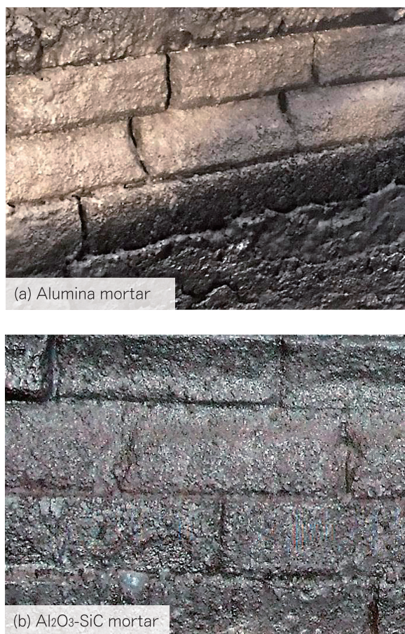
Fig.4 Hot faces of Al 2 O 3 -SiC bricks in actual tundish after use for about 30 charges; (a) installed with alumina mortar, (b) installed with Al 2 O 3 -SiC mortar.
