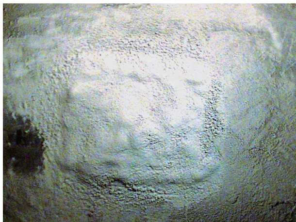
Fig.7 Structure appearance of gunning material LX-160G-1 application test.
