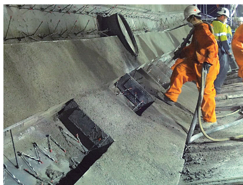
Fig. 6 Installation of NOVACRETE shotcrete into a rotary kiln.
