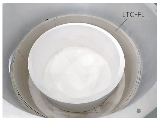
Fig. 4 Appearance of LTC-FL relined in cylindrical furnace.
